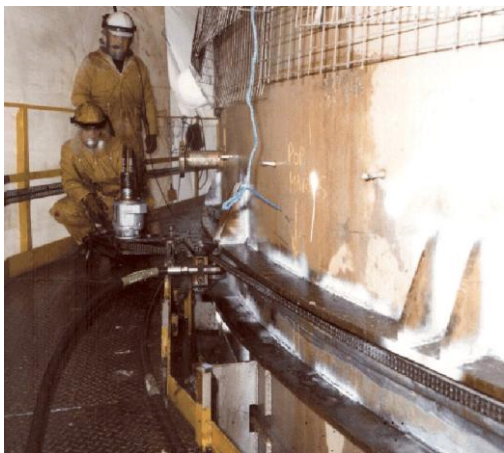
Decommissioning of storage tanks
