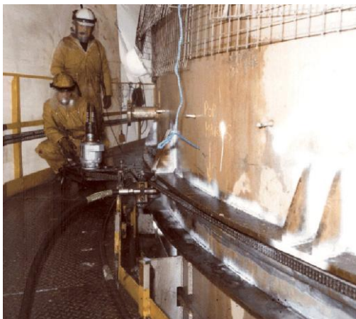
Decommissioning of storage tanks
